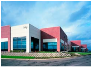
CENTRAL PLANT 1-2 million liters of UPW/day
